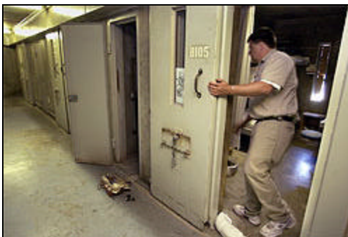
Plumber Brian Coughran changes a water valve in a cell at California State Prison, Sacramento, where the sewage and water system has frequent breakdowns and vandalism. Prison plumbers are classified as public-safety workers, making them eligible for fatter pensions and disability benefits.
